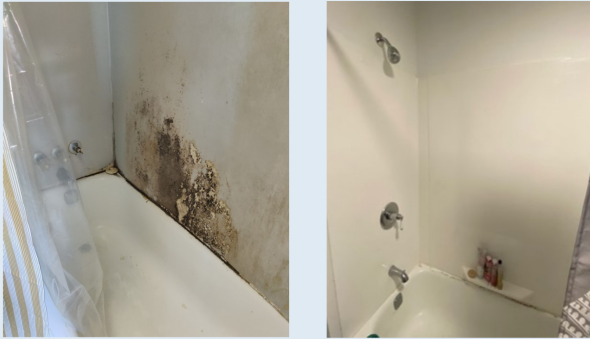
Moldy Bathroom Surround Replaced
