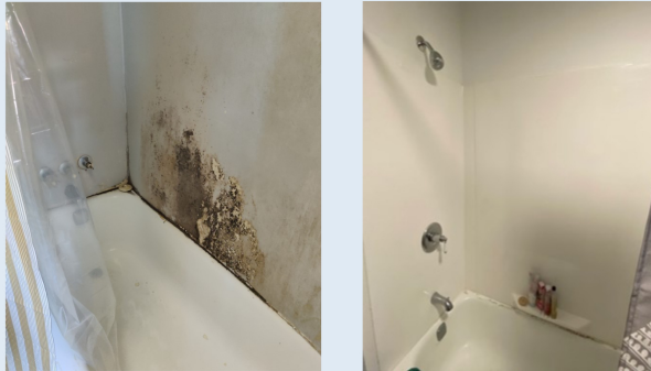
Moldy Bathroom Surround Replaced
